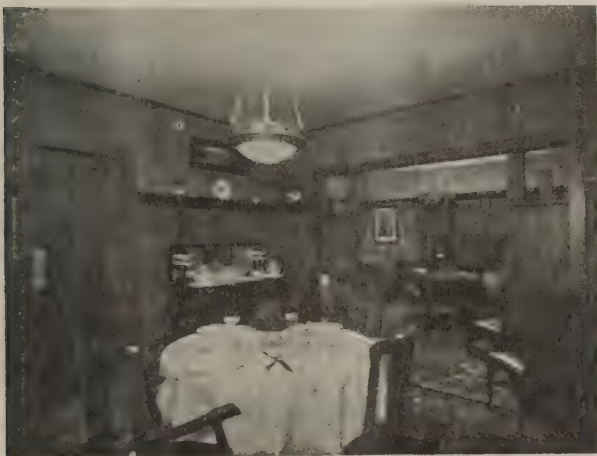
Fig. 1. The semi-indirect unit illuminates the dining room too uniformly and the ceiling is too bright compared with the table
